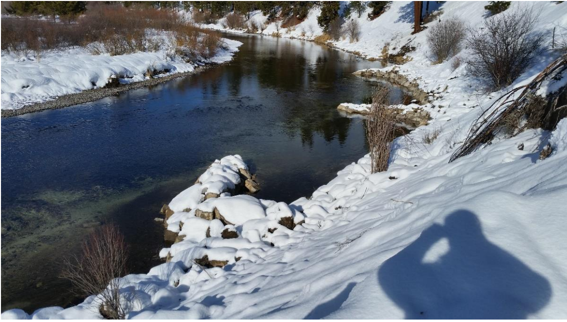
Figure 6. Installed Rock Barbs
