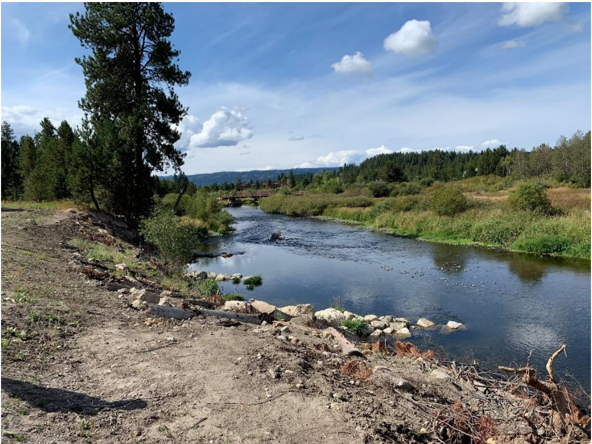
Figure 7. Installed Rock Barbs
