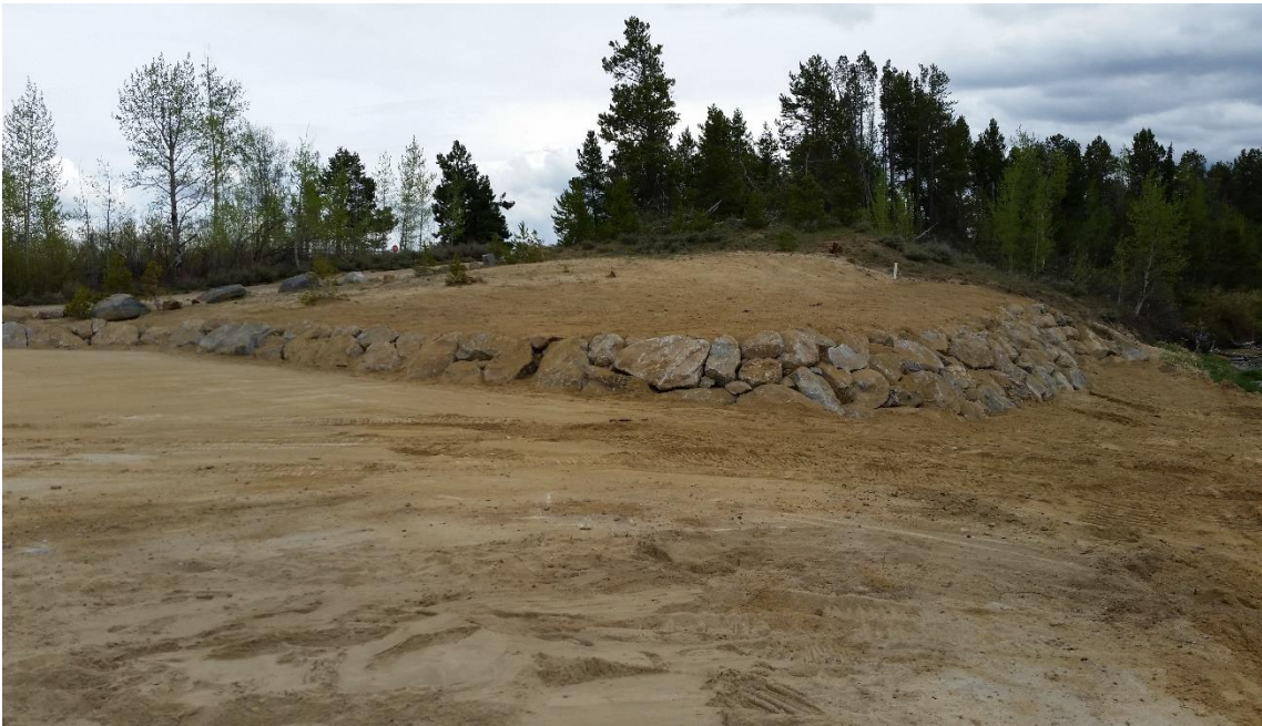
Figure 3. Newly Constructed Retaining Wall
