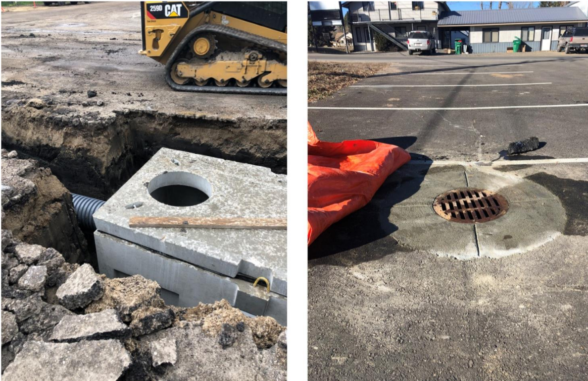
Figure 12. Installation of and Completion of Grease Interceptor
