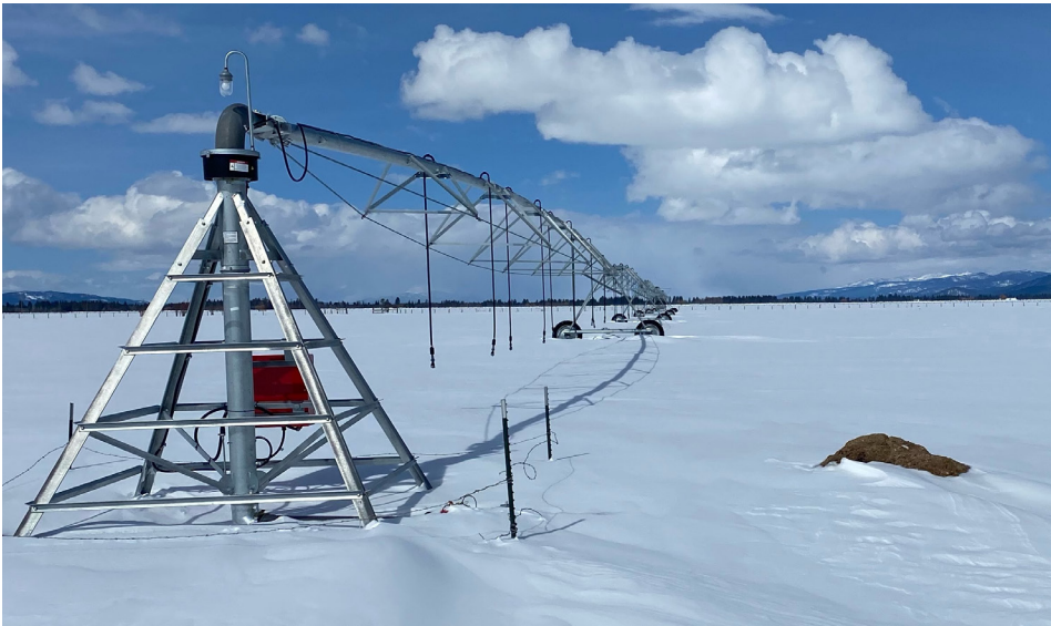
This is one of four pivot irrigation systems installed in 2022 via Idaho DEQ Ag BMP grants. The pivots will reduce sediment, phosphorus and nitrogen flows into Lake Cascade. (courtesy Valley SWCD)
