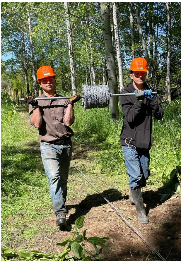
Idaho Conservation Corps workers roll out wire for the riparian fencing project (courtesy Valley SWCD).
