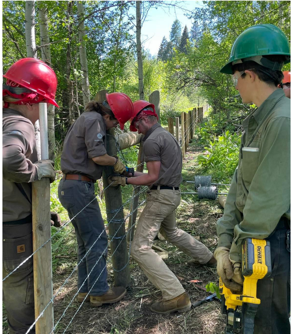
Members of the Idaho Conservation Corps install riparian fencing to keep livestock and ATVs away from lakeshore areas (Courtesy Valley SWCD).
