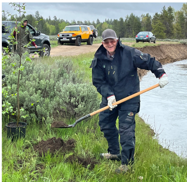
Lenard Long digs a hole for a new shrub to help anchor the streambank (courtesy Valley SWCD).
