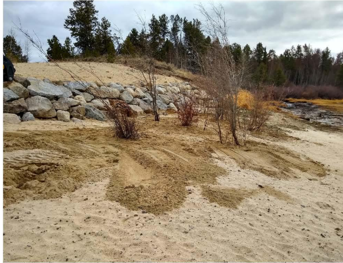
Newly planted willows should help reduce the flow of sediment to the Lake.
