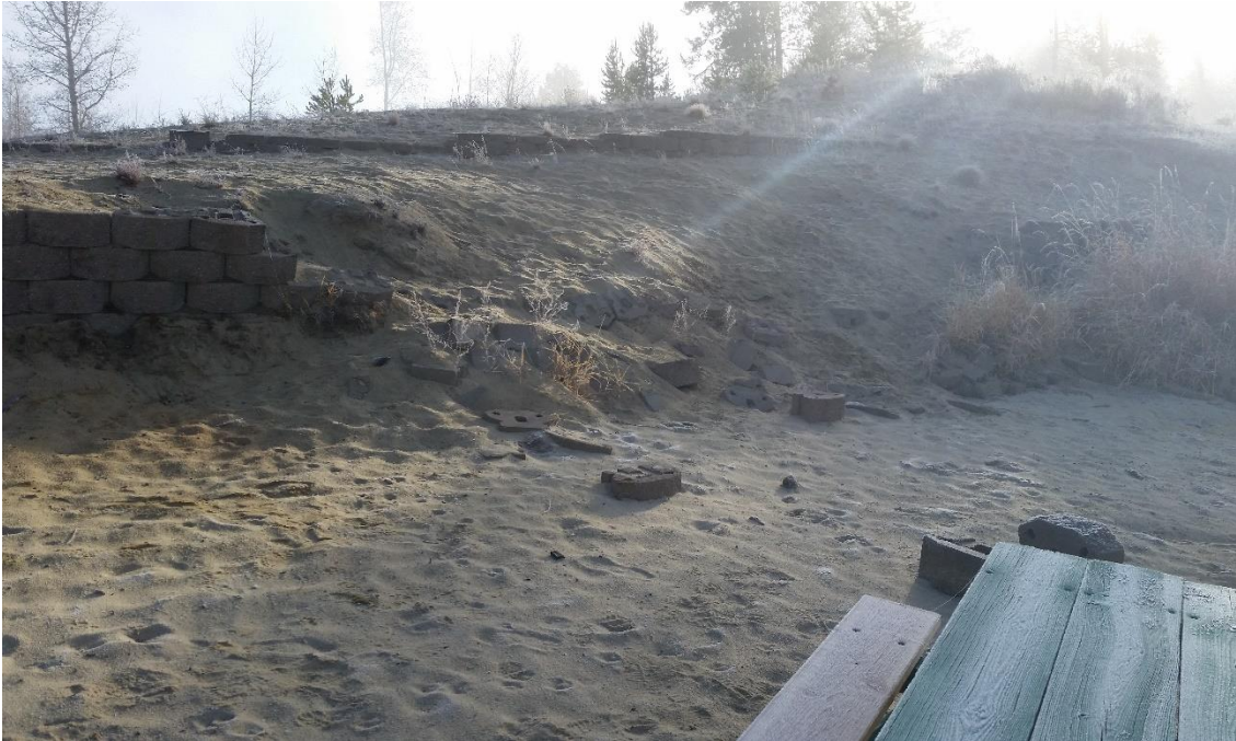
Figure 2. Old Retaining Wall
