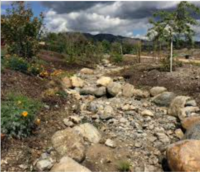
Vegetated Bioswales Filter, slow down, recharge stormwater
