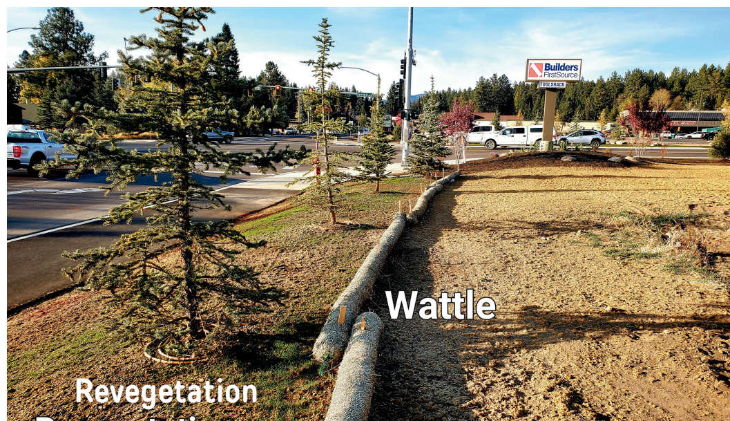
Other siltation control measures - commercial site
