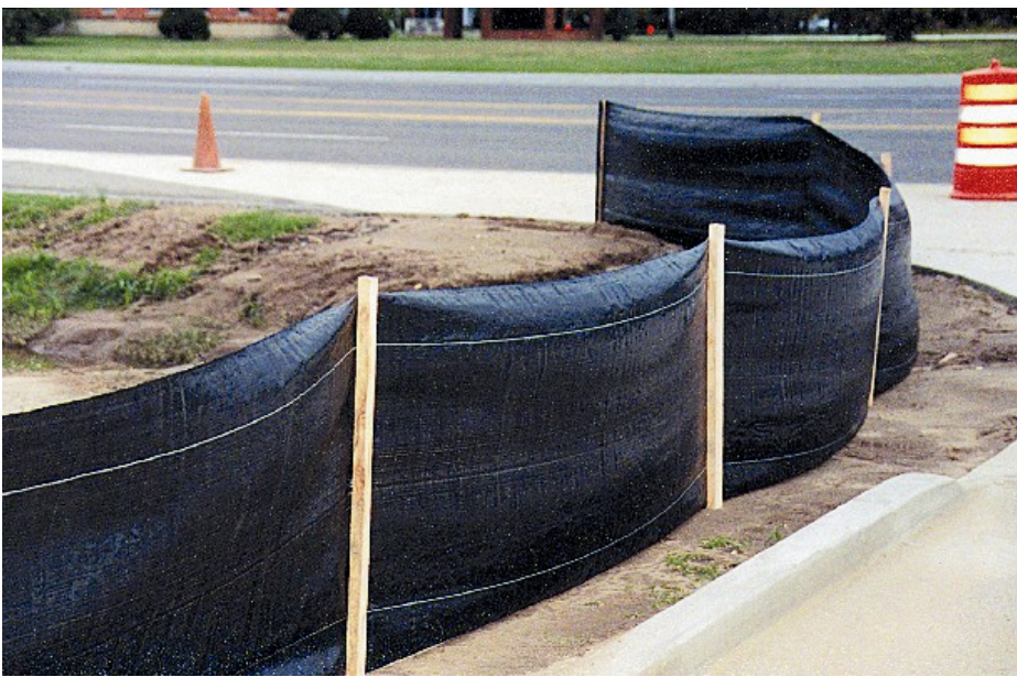
Silt fencing to control erosion into waterways
